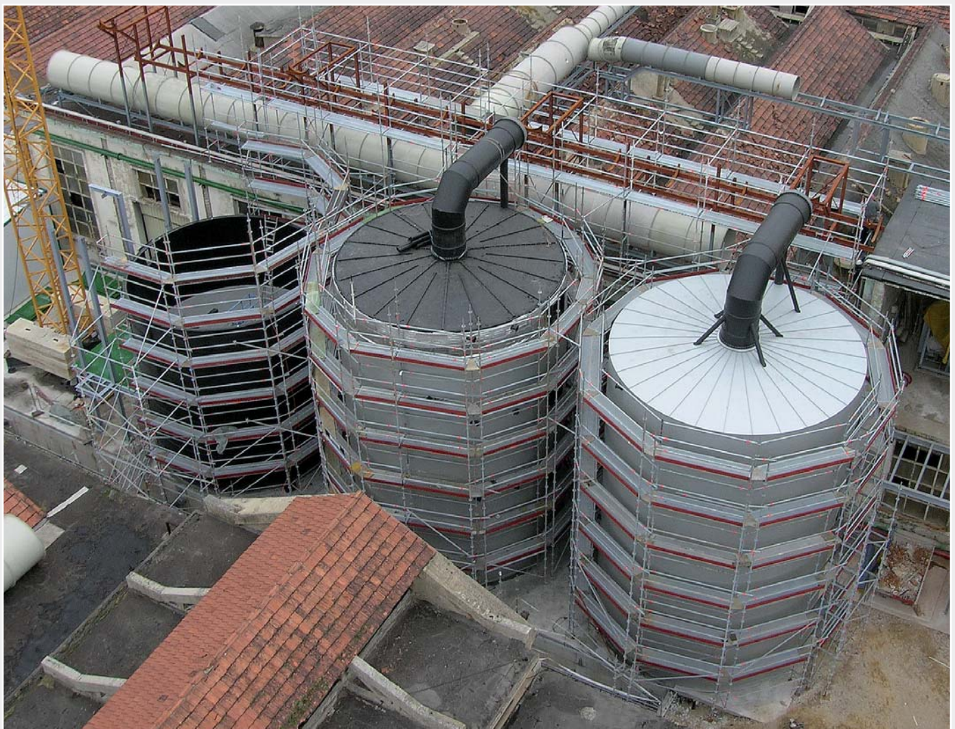
The almost completed silos prior to connection with the cellulose factory.
