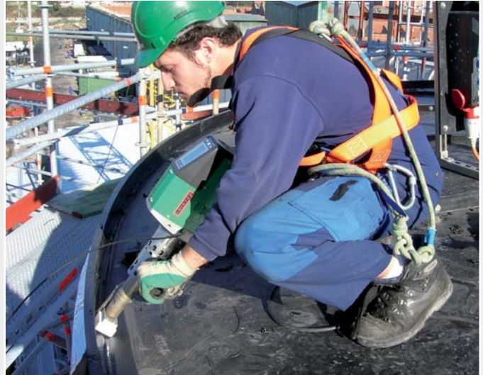
Connecting the wall and roof elements in Spain with a WELDPLAST EC 4.
