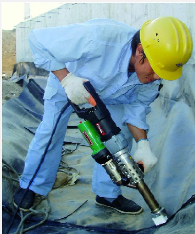
**Extruding the sealing sheets on uneven subsurface with the FUSION 3 hand extruder.**
