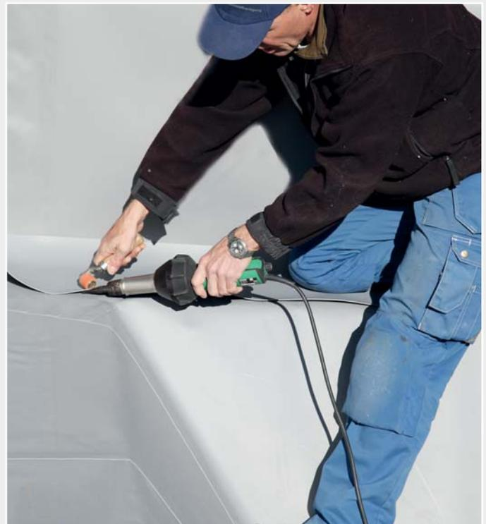
*The handy TRIAC AT allows welding in hard-to-reach places like here on the edge of the pool.*
